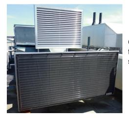
On the front of every AHU is a grille (or Air Intake Screen) to prevent large, unwanted objects from entering the system and potentially causing damage or a blockage.
