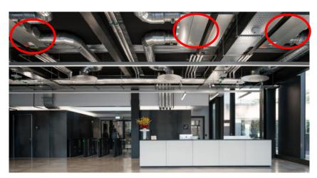
The image to the left shows several exposed FCUs, providing this office foyer with heated/cooled air.
