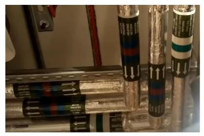
Each pipe will be colour coded (depending on whether it is heating (red & blue) or chill (green)) and will also have arrows indicating the direction of the water.
