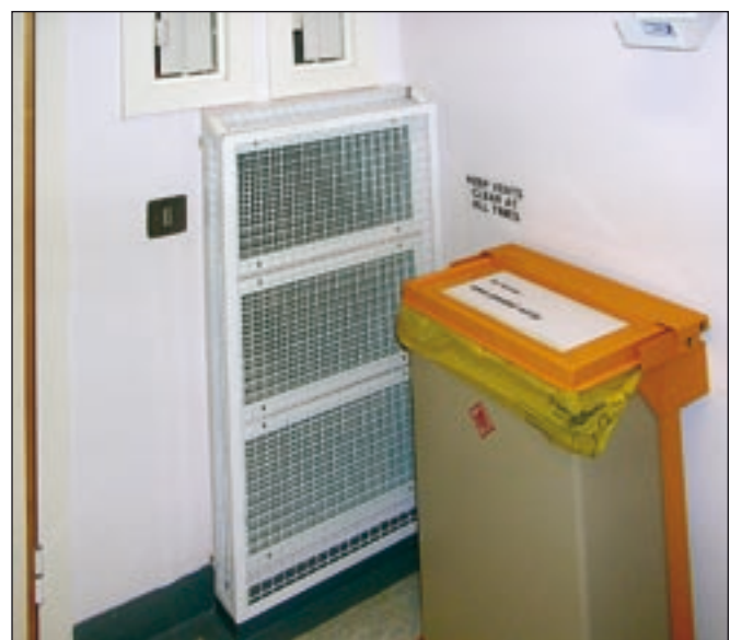
Pressure stabiliser with stand-off cage
