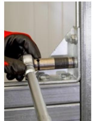
Finally, using a calibrated torque wrench tighten all the screws to the torque value specified in the MX Technical Book.
