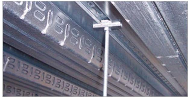
There are several metal deck systems each with slightly different profiles and slots, and it is important to use the corresponding wedge nut.
