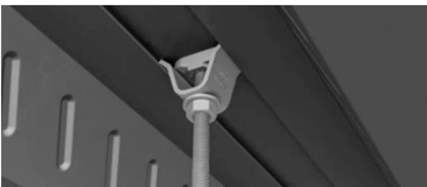
The wedge nut is locked by tightening the nut against the locking plate.
