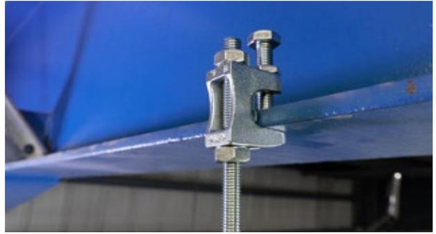
Parallel Steel Flanges – the beam clamp can be installed either way up.
