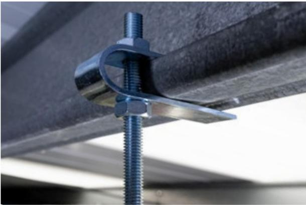
Safe loads that can be applied to the purlin flanges are relatively low and often no more than 15kg -20kg depending on the size of the purlin. When approved, purlin clips should only be used for lightweight services and the clips must be adequately spaced to prevent overloading the purlin flange.
