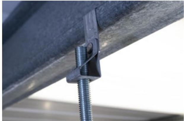
Manufacturer's published loads for spring steel purlin clips can be misleading. These are safe loads for the clips and do not consider the maximum load for the purlin flange. The smaller of these two loads applies to the suspension.
