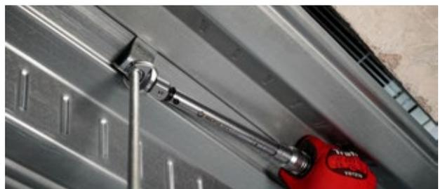
**IMPORTANT** – to achieve the design load it is important to tighten the nut to the manufacturer’s specified torque value.
