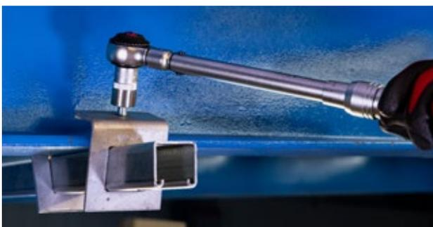
Tighten the bolts or nuts to the torque value specified in the MX Technical Book. This is especially important for cone-pointed screws which bite into the surface of the steel. These are liable to be overtightened which reduces the clamping strength of the connection.
