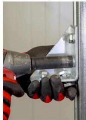
Using a cordless impact wrench speeds up the installation and helps maintain alignment of the brackets during tightening. The impact wrench must be set to tighten the screws to less than the final torque requirement.
