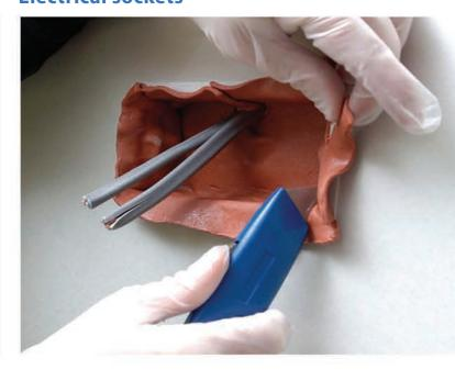
When electrical outlets (back-boxes) are fitted into partition stud walls they must be fire-stopped to prevent fire penetration through the plasterboard and into the cavity using an intumescent based pad.
