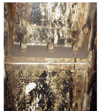
Tunnel ring caulking
