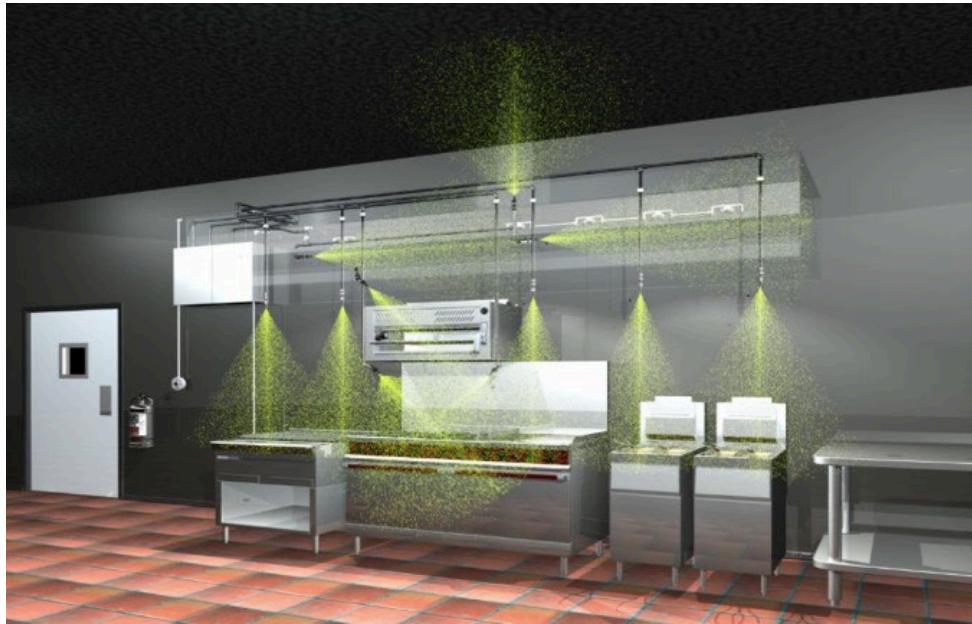
Example of a Fire Suppression System
